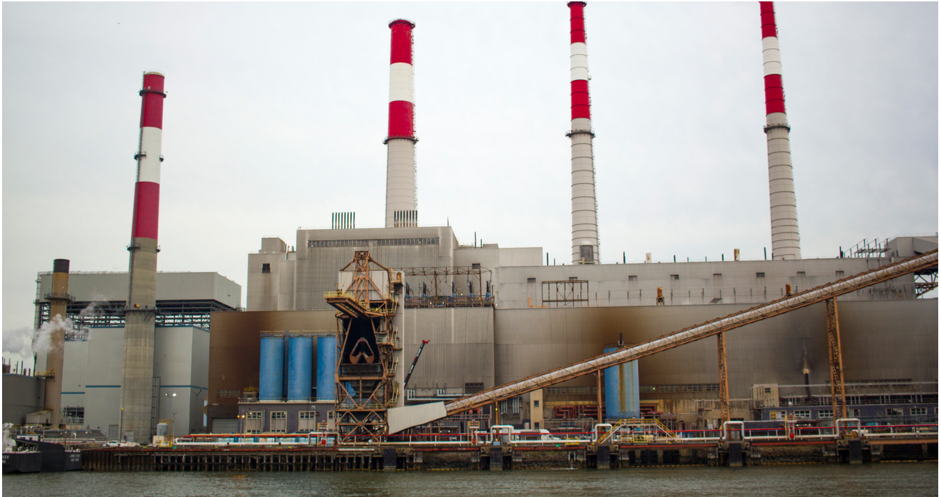
Ravenswood Generating Station in Long Island City, Queens, New York. PHOTO: iStock
