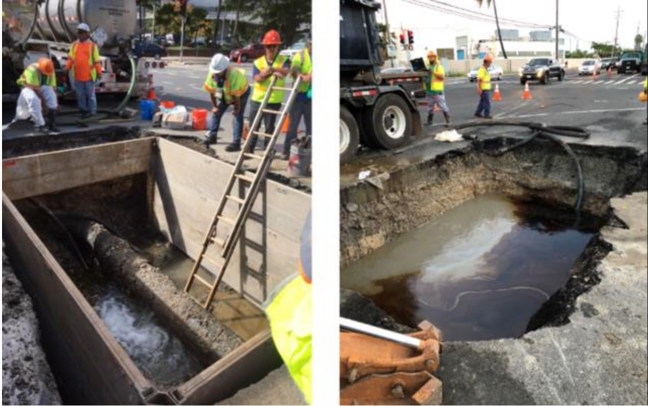
Figure 9: Water Main Repairs at Intersection of Nimitz and Alakawa, July 2018
