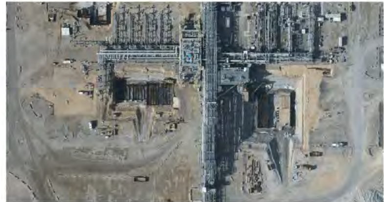
Field facilities: anchor blocks at 3GI
